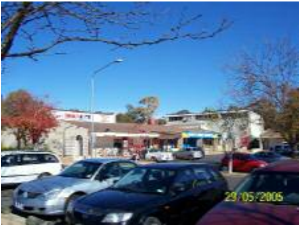
Area C shops from inside Rivett Place near Area D on Outcome Drawing
