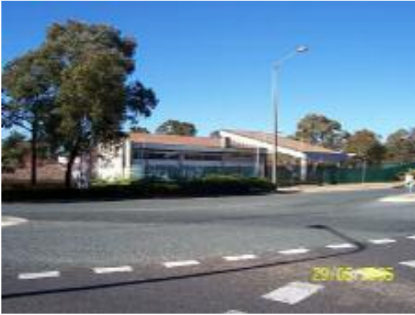
Disused Service Station from the intersection of Angophora Street and Bangalay Crescent
